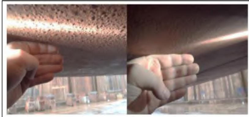
Figure 16 – Comparison of surface quality in regions where abrasive blasting has been applied (on the right) and where no abrasive blasting has been applied (on the left)
