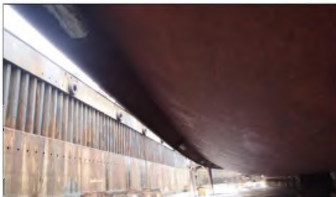
Figure 13 – Zinc anodes on the portside bilge keel
