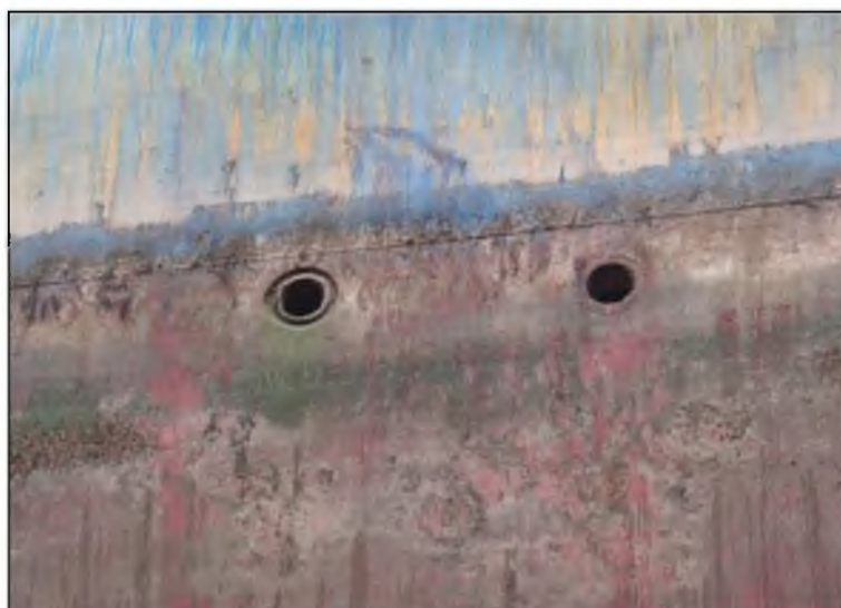
Figure 12 – Hull openings at starboard side midship
